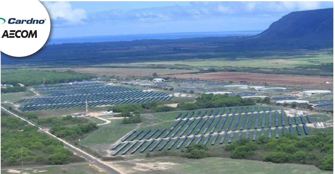
Above: US DOD's Pacific Missile Range Facility includes a 14 MW solar facility paired with a 70 MWh battery energy storage system. Image credit: Cardno and AECOM ©
